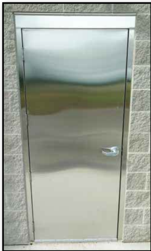
SS DOOR IN CHANNEL FRAME
