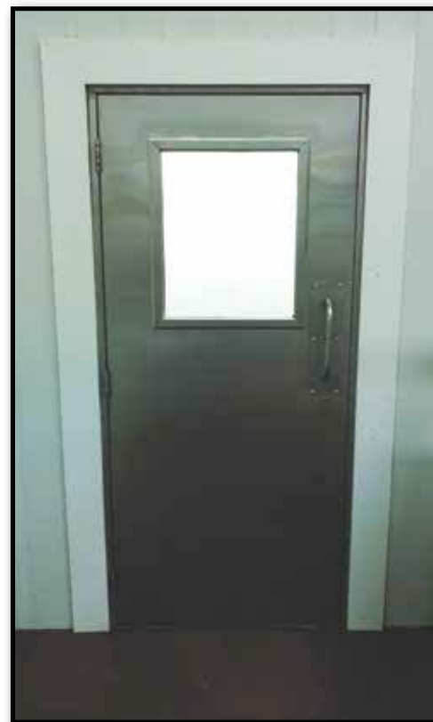
SS DOOR IN CHANNEL FRAME
