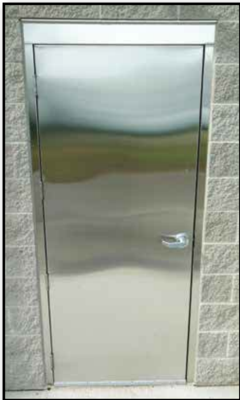
SS DOOR IN CHANNEL FRAME
